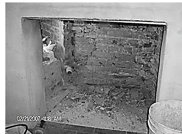
Badly Deteriorated Firebox
