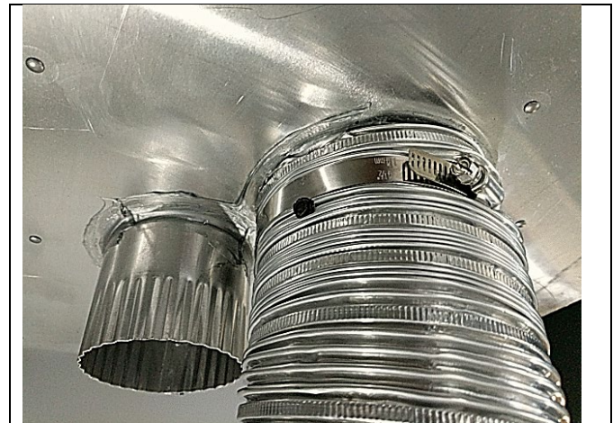
Vent Cap Flex Connection
