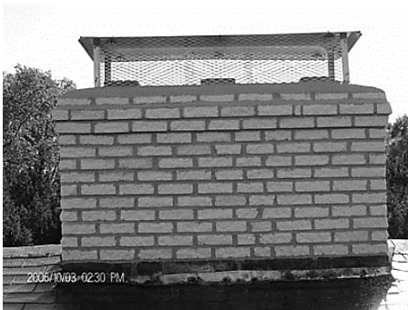
Metal Cap on Clay Liner Chimney Top
